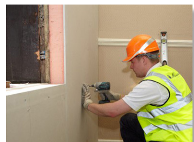
3. Internal Wall Insulation
